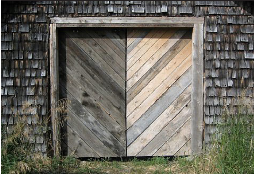
A pickling solution has been applied to the door on the left.
