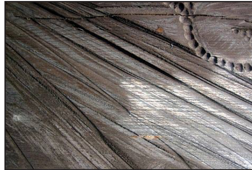
Wood that has been "pickled"
